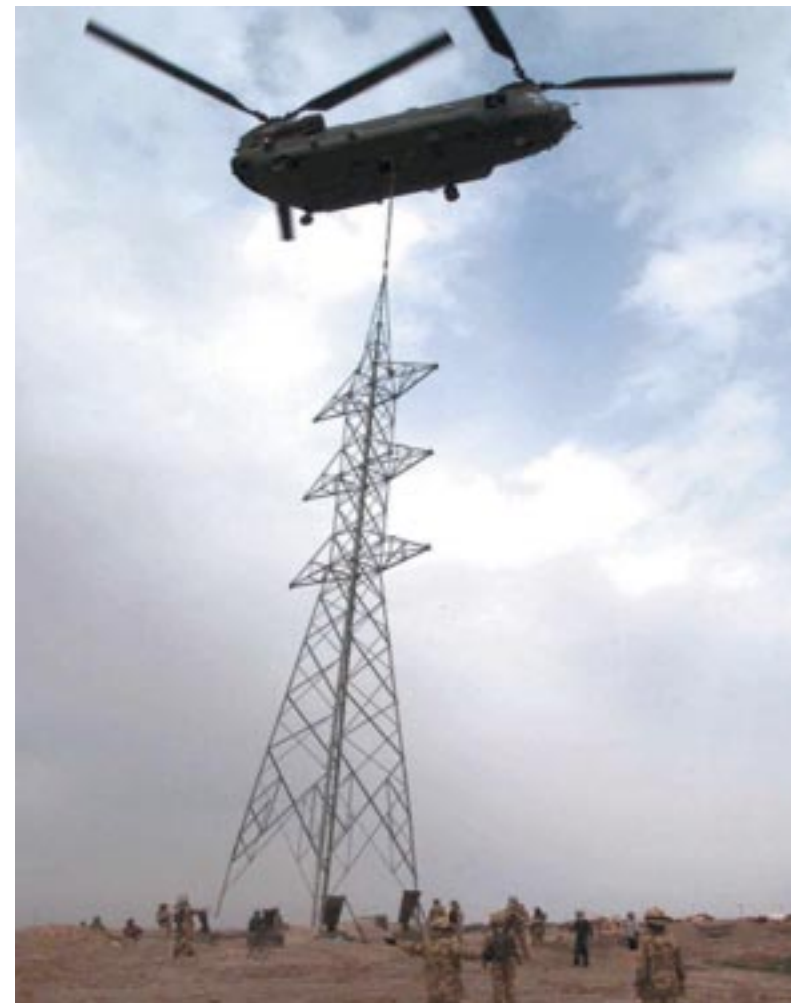
Infrastructure repair in Iraq
